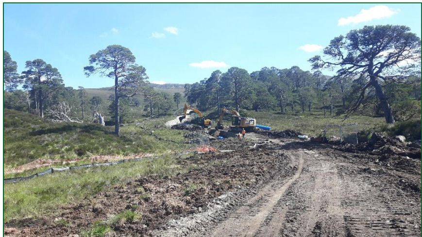
Pipe laying at Allt Garbh.
