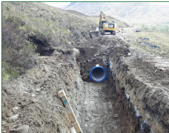
Penstock pipelaying nears completion
