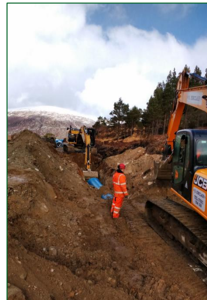
Penstock – work progressing.
