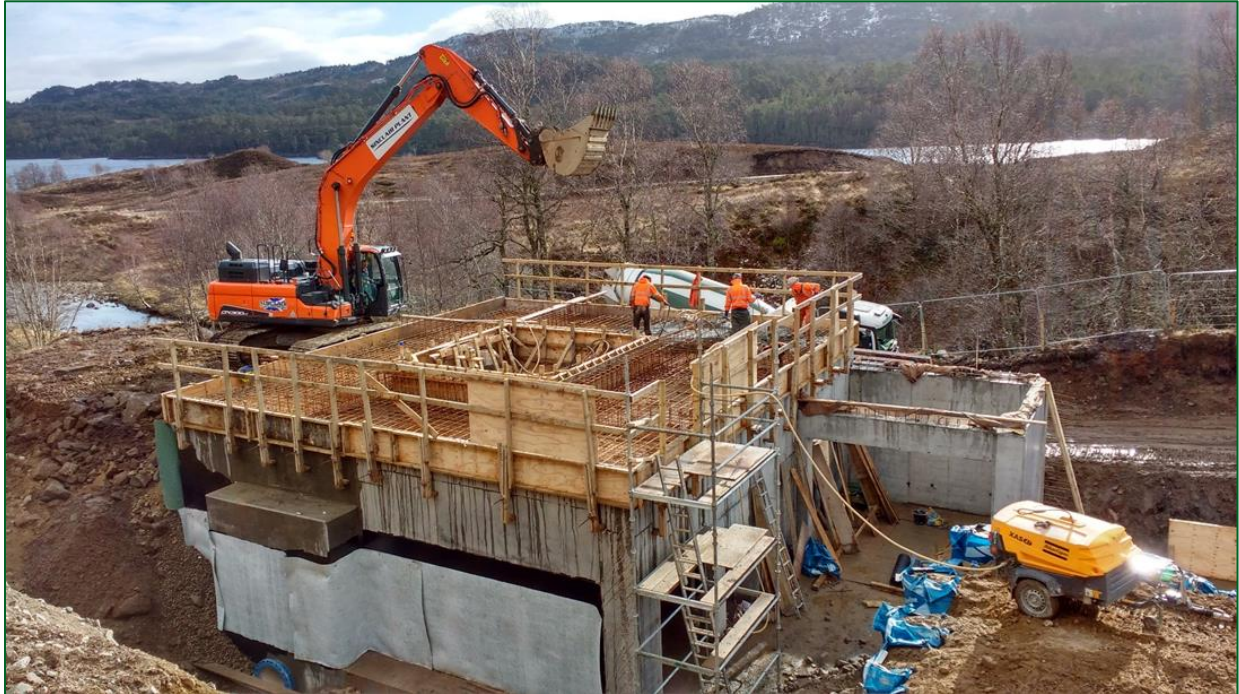
Abhainn Gleann nam Fiadh powerhouse – roof slab concrete being placed.
