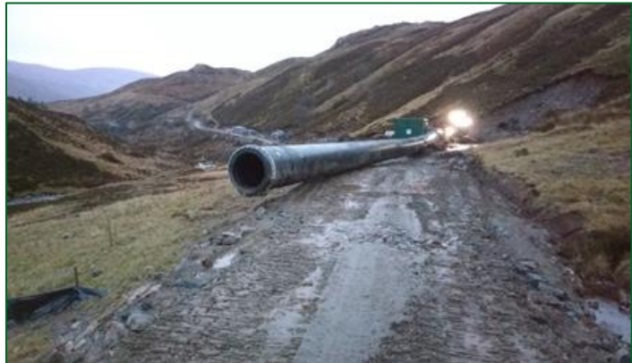
Alt Garbh – upper penstock pipes being welded
