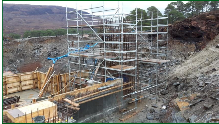
Alt Garbh powerhouse – Rebar being fixed for thrust block
