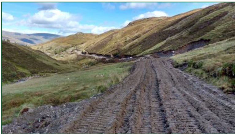
Allt Garbh – access track complete to the intake (left).
