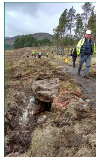
Works ongoing at the new footpath
