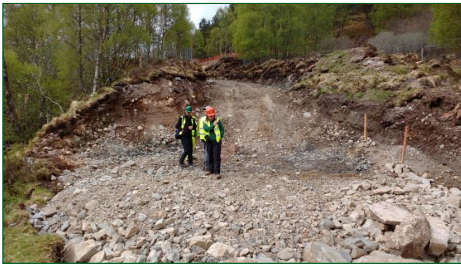
Outfall – Bulk earthworks complete.
