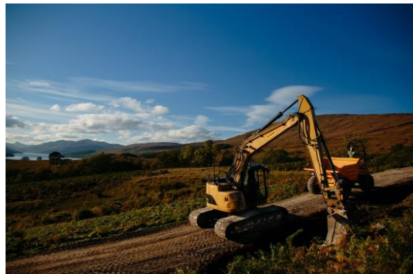
Example of penstock access track – Loch Arkaig
