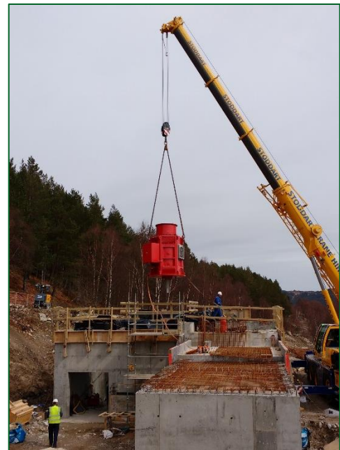
Turbine installation, Abhainn Gleann nam Fiadh.
