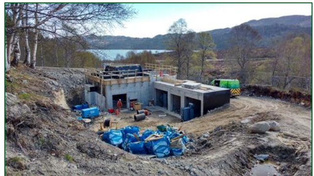
Powerhouse – now structurally complete.
